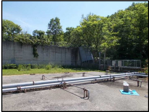
堰堤 (浸出水出口側)
